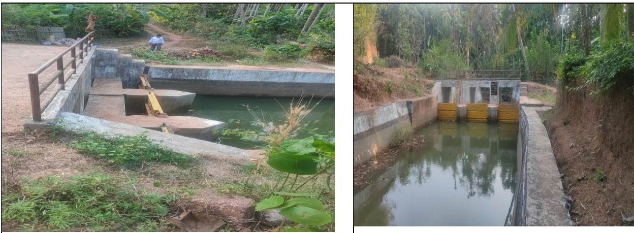
Figure 23: Field Photographs of Vented Dams
