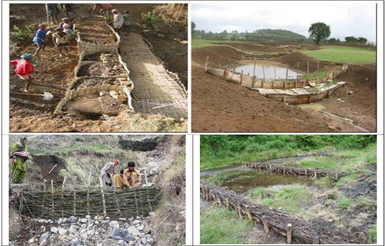
Fig 48 : Gully plugging works
