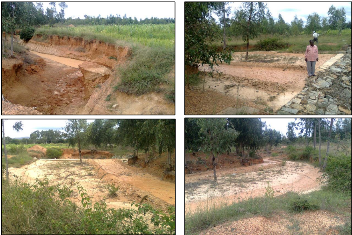
Figure 24: Photographs: Check Dams without periodic maintenance
