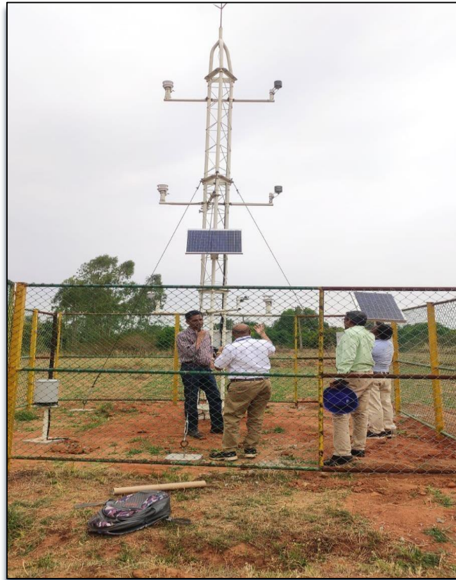
AMS Tower Installed in the Field
