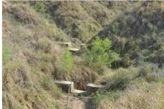
Ravine Reclamation Structure
