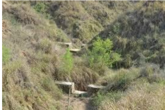
Ravine Reclamation Structure
